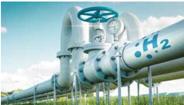
Sealing of Gas Tanks and Pipes
